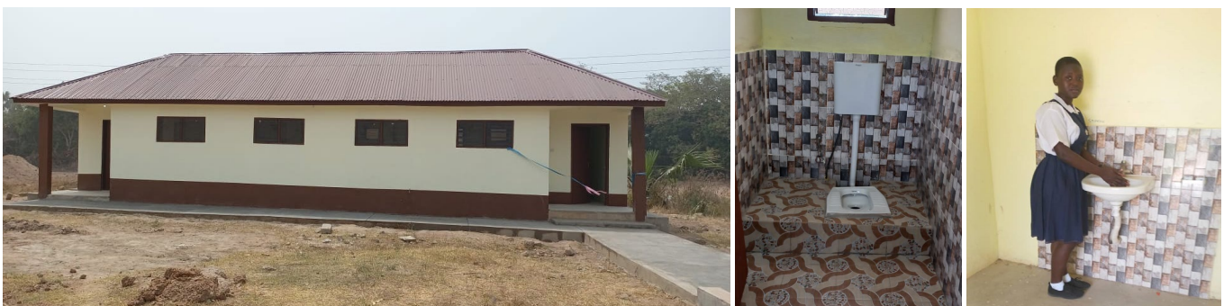
[foto's: project 2022-1-10 van St Ann Girls Senior High School – de 8 bio-digester toiletten]
